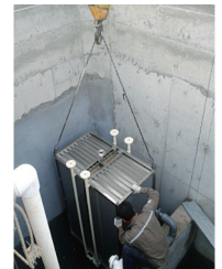
Wastewater treatment MBR membrane module (Taiqinggong, Laoshan)
